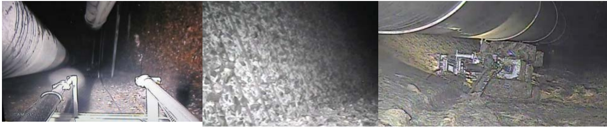
Fig. 1: Images from inside the CAEX Tunnel: (left) a view from the 2015 Recover Crawler (RC), (center) a close up of the deterioration of a tunnel wall, and (right) an image of the tipped over 2014 Inspection Crawler (IC) in the muddy debris under a duct. [1]
