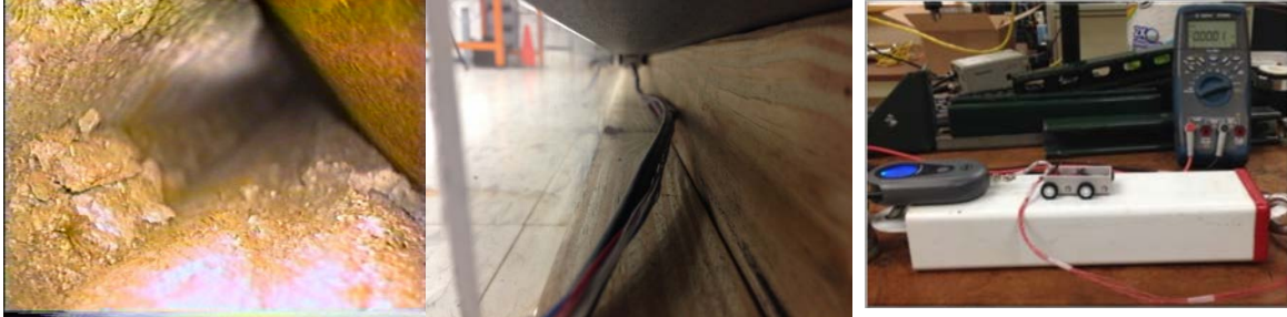
Fig. 9: Debris in refractory air slots, mock-up test bed and maximum pull force testing.
